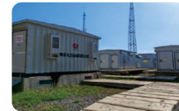
Yuncheng Power Plant: Peak Shaving Project
